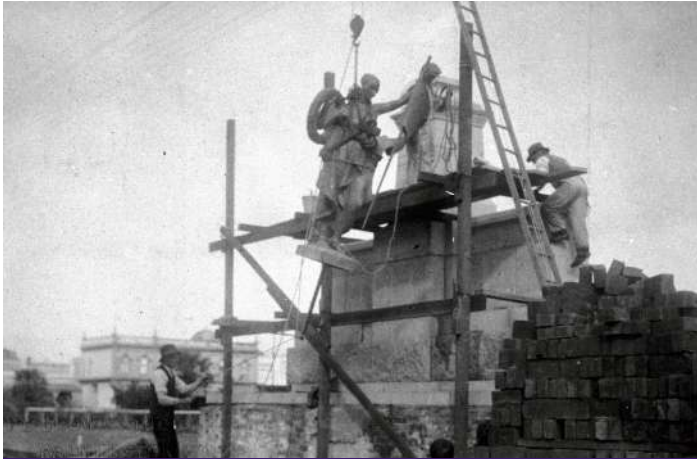
The bronze ‘Spirit of Motherhood’ statue being raised in place on the Palmerston North War Memorial, c. 1926. Photo / Manawatū Heritage
