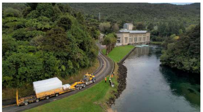
The picturesque Tuai Power Station site. Photo / Genesis Energy
