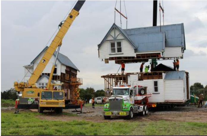
St. Matthew's Vicarage in some of its various sections for the move. Photo / Chessa Stevens
